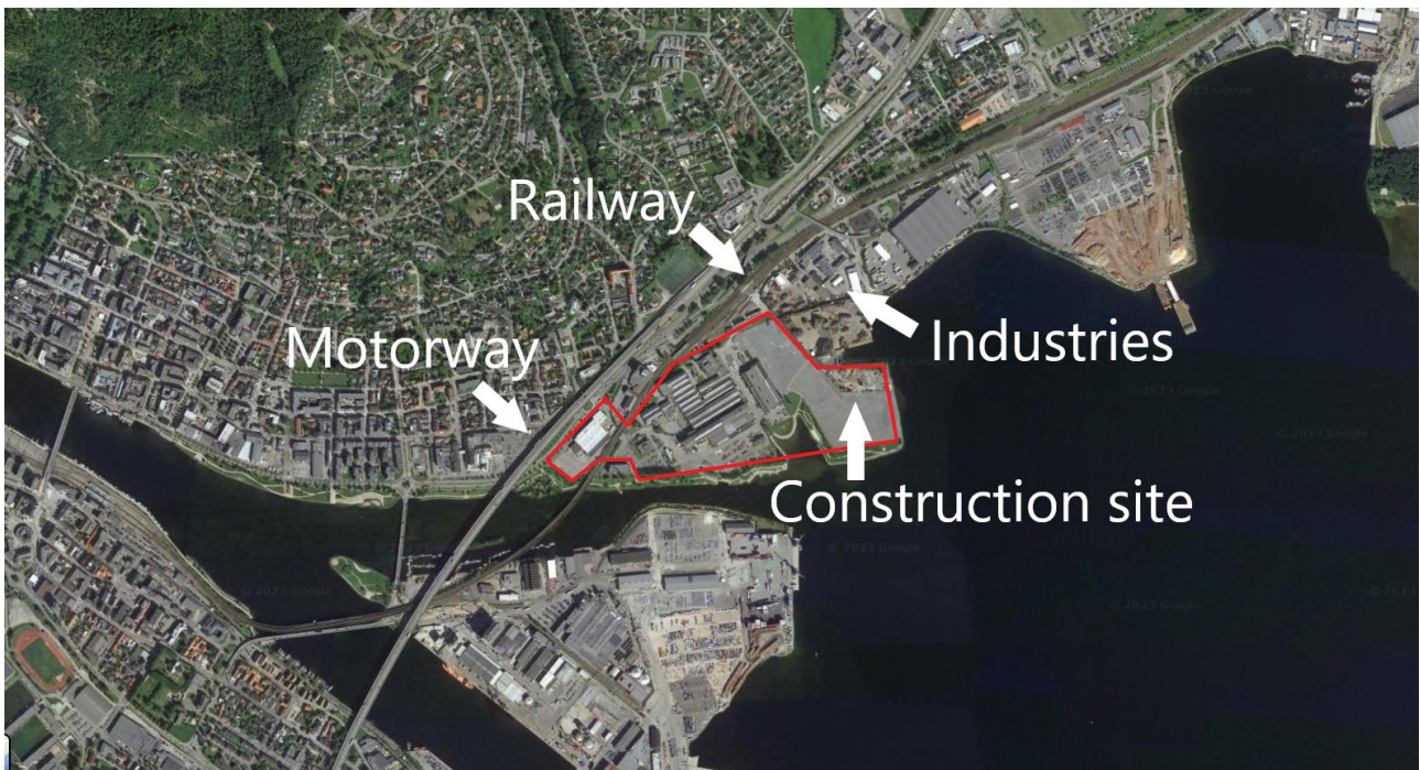
Figure 5 - Construction site in a complex urban soundscape. The construction site of the new Drammen Hospital is marked in red. Residential areas are located to the left side of the motorway.
